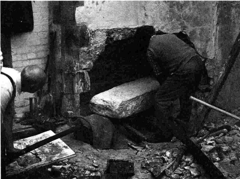
Iken: removing the cross-shaft from the base of the tower.
